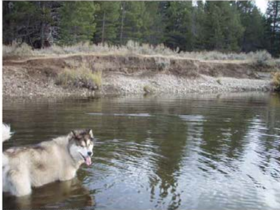
Eroding Bank at RS 10000
