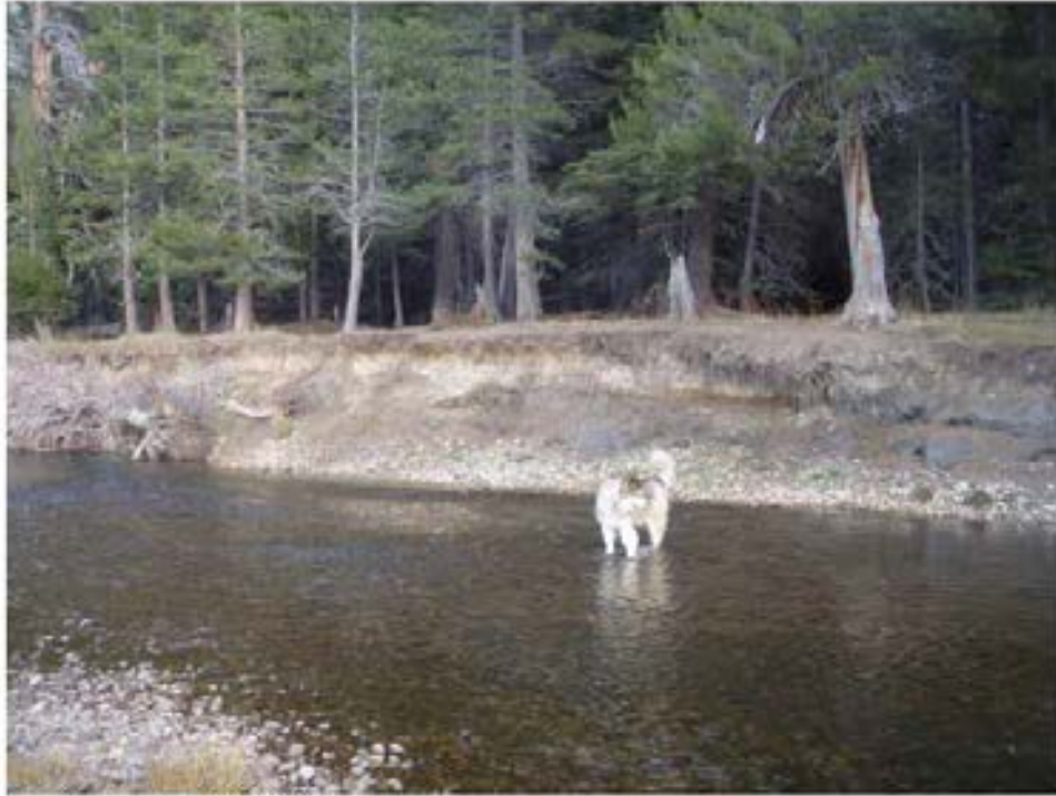
Eroding Bank at RS 9300
