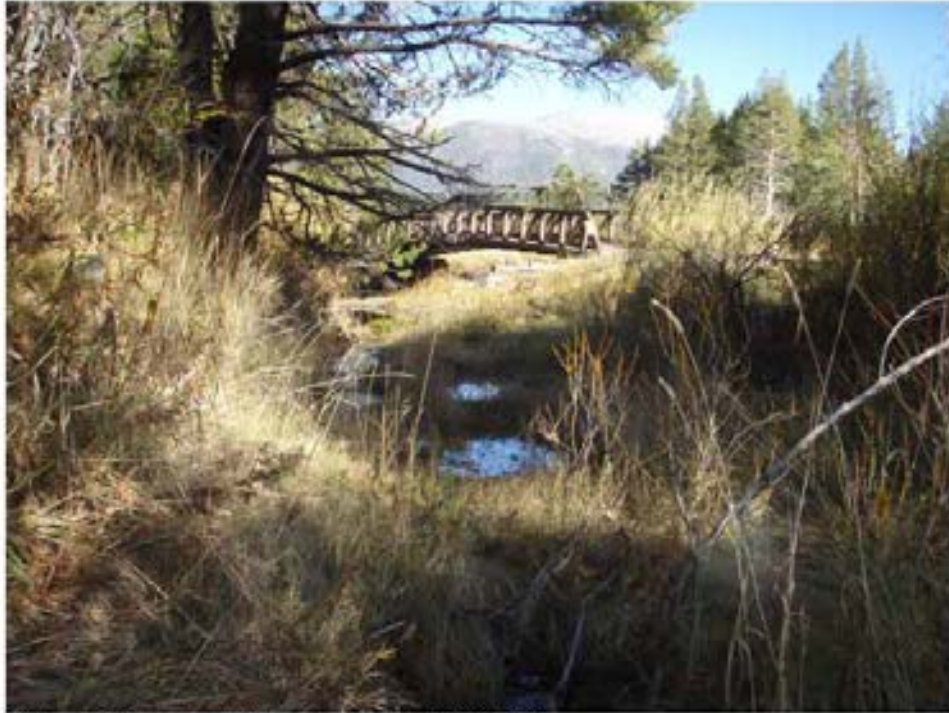
Historic Channel at Bridge for hole #7 RS 7600
