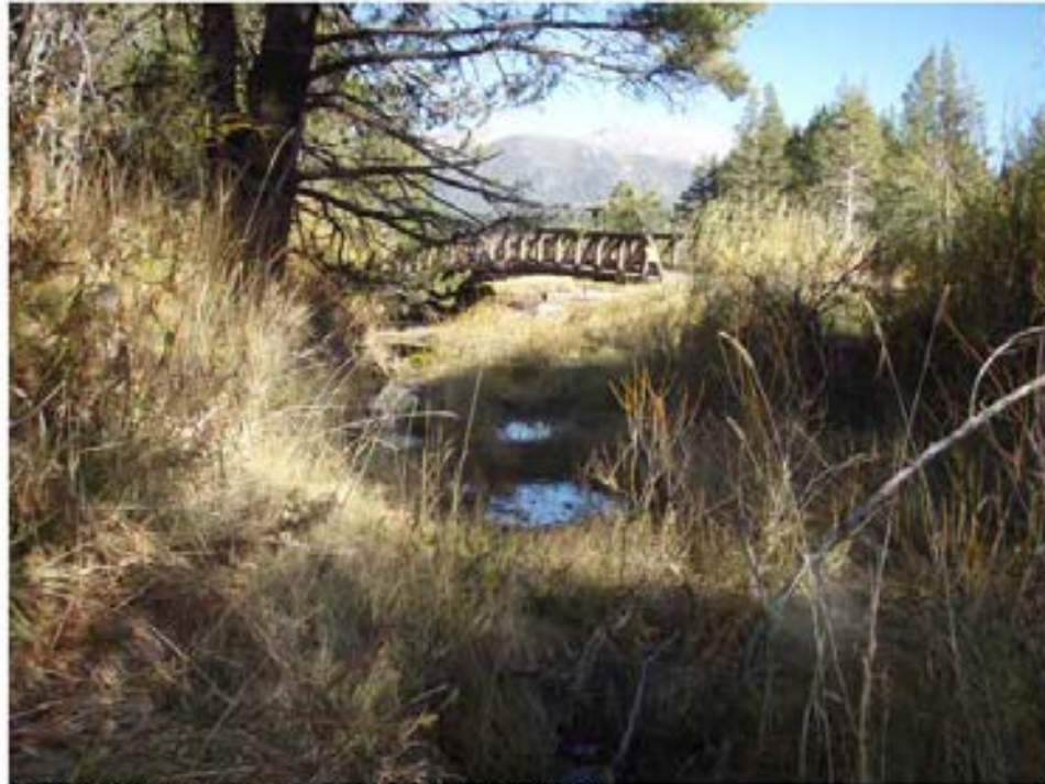
Historic Channel at Bridge for hole #7 RS 7600
